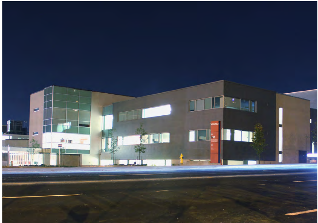
1.14 IMAGE: BUILDING “A” ADDITION REALIZED AT NEWNHAM CAMPUS
