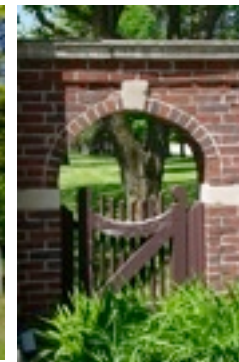
.37, .38 Entrance gate wing wall and gateway to the house. Note the man door gateway detail.
