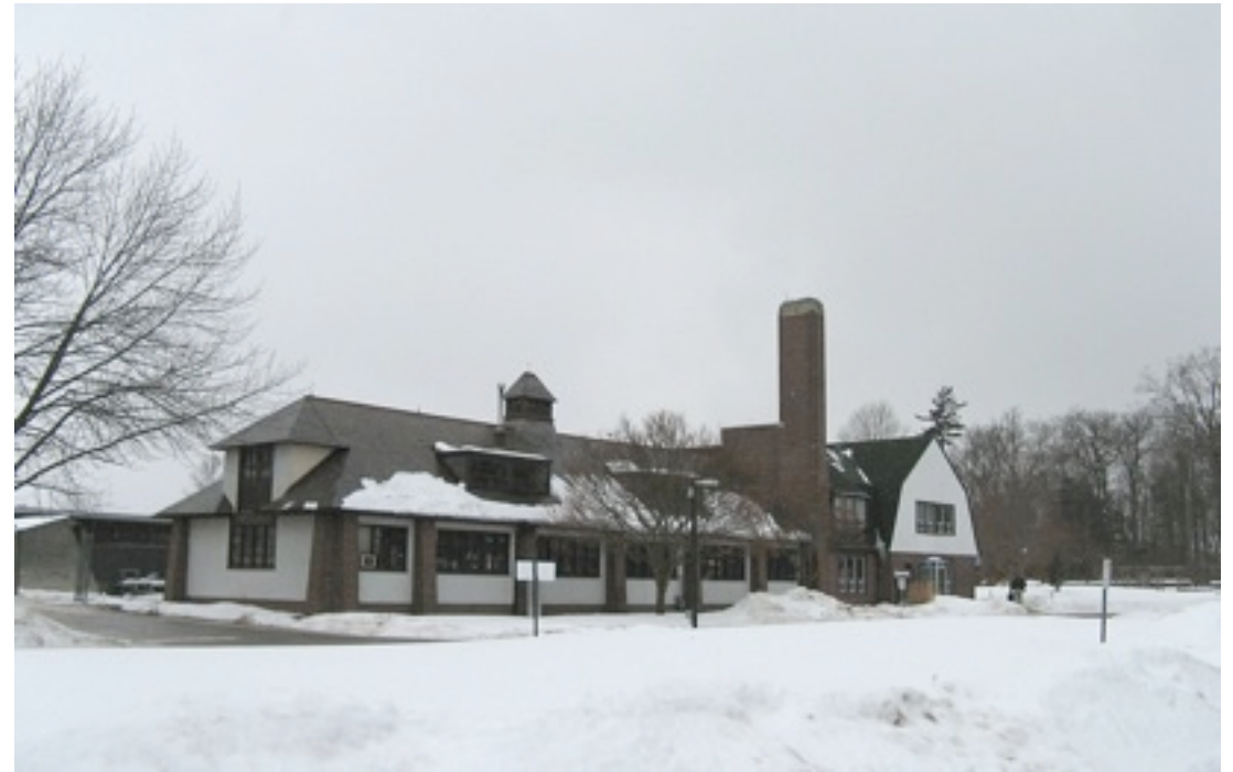
17. The Eaton Dairy Barns
