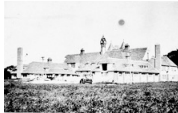
.10 Historic Image of the Eaton’s dairy farm complex c. 1920s. The buildings at the right front can survived a devastating fire that took the main barn in the 1960s. See below.
