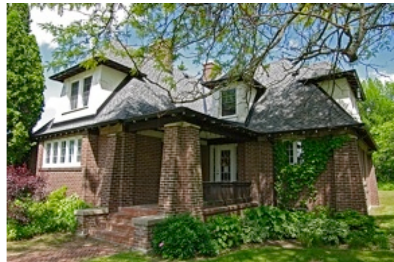
.39 View of gate house from the SE. The entrance porch and doorway are in alignment with the gate posts in the wing wall pictured above. It is a charming and picturesque Arts and Crafts design.
