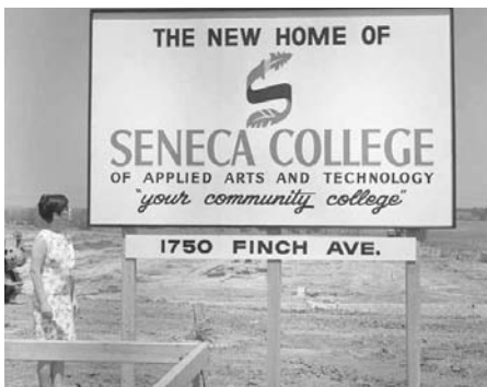
A sign in 1968 marks the future location of the Newnham Campus
