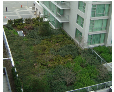
The Campus Master Planning Process presents an opportunity to demonstrate leadership in sustainable design
